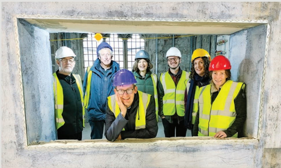
The Revd Phil Medley (front centre) joins project leaders and diocesan representatives as they look through what will be a new serving hatch
