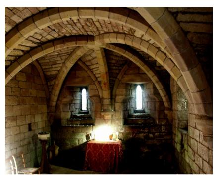
Five steps lead down from the south door to the slabbed floor of the main crypt chamber, which has a groined vault in two bays: the NCH (107) describes it as being 'a peculiar combination of quadripartite sexpartite forms, the outer halves of each bay being of the latter, which the inner, where they conjoin, is of the former construction. transverse rib semi-circular'. The vault ribs are all chamfered on their lower angles. Three lancets that light the crypt -
