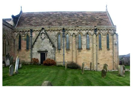
Chancel The is constructed of yellowish coursed squared stone; there has been extensive restoration and re-facing. It is five bays long, and has a large plinth with a bold roll at the top and chamfered below. The second bay the from west remodelled in the early 19<sup>th</sup> century, and has a priest's door set in a shallow gabled projection, of grey
