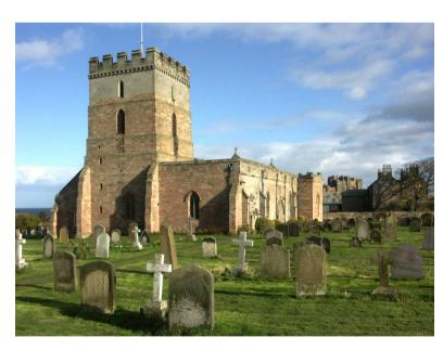
The only sections of the **Nave** walls exposed externally are above the aisle roofs, and the eastern gable; all these are clearly 19<sup>th</sup>-century fabric, of elongate blocks of grey stone, and are capped by moulded copings, with a finial cross on the gable.
