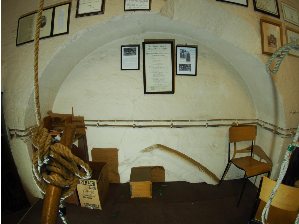
The east side of the Ringing Chamber, with the head and hoodmould of the 13 th century east window, within a rough semicircular arch of the same date, which probably carried a bellcote.
