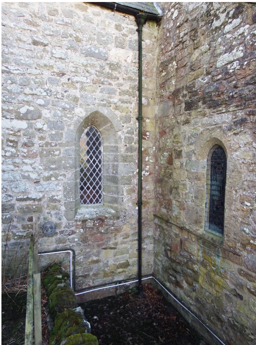
The north wall of the chancel with its low-side window, and east end of the north aisle with a genuine 13 th century lancet
