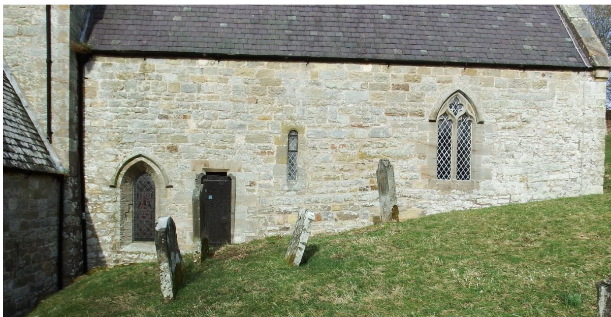
The south wall of the Chancel
