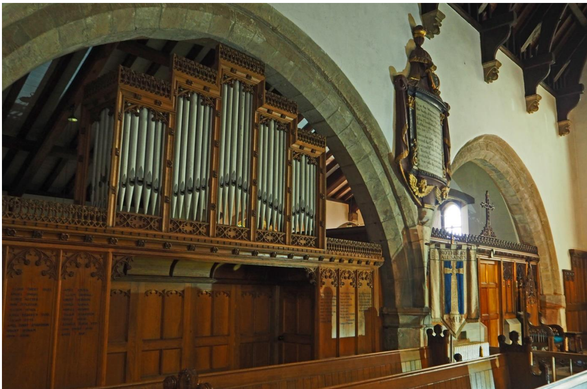
North chancel arcade, formerly opening into Cartington Chapel
