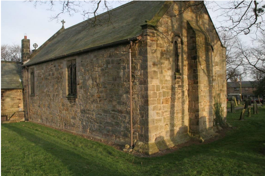
The nave from the north-west
