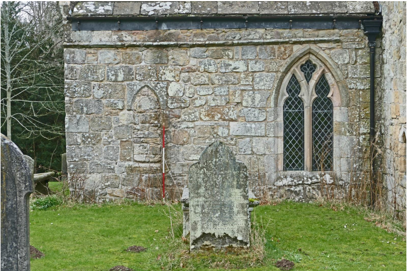
The South Chapel, east wall.
