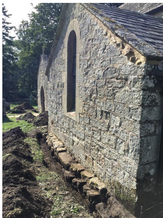
South end South Transept with footings
