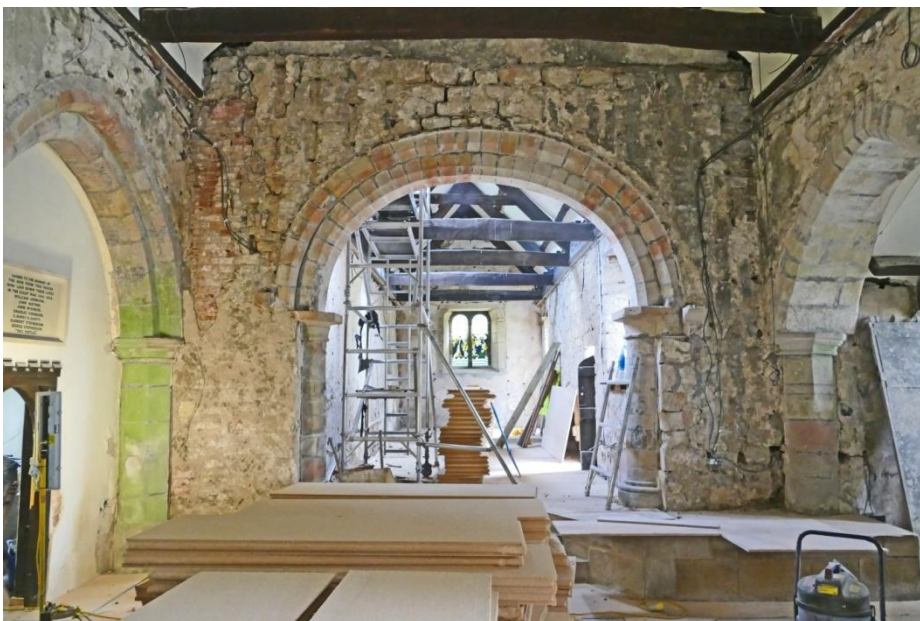
Interior looking east during the 2018 works, showing chancel arch, and eastern respond of south arcade.
