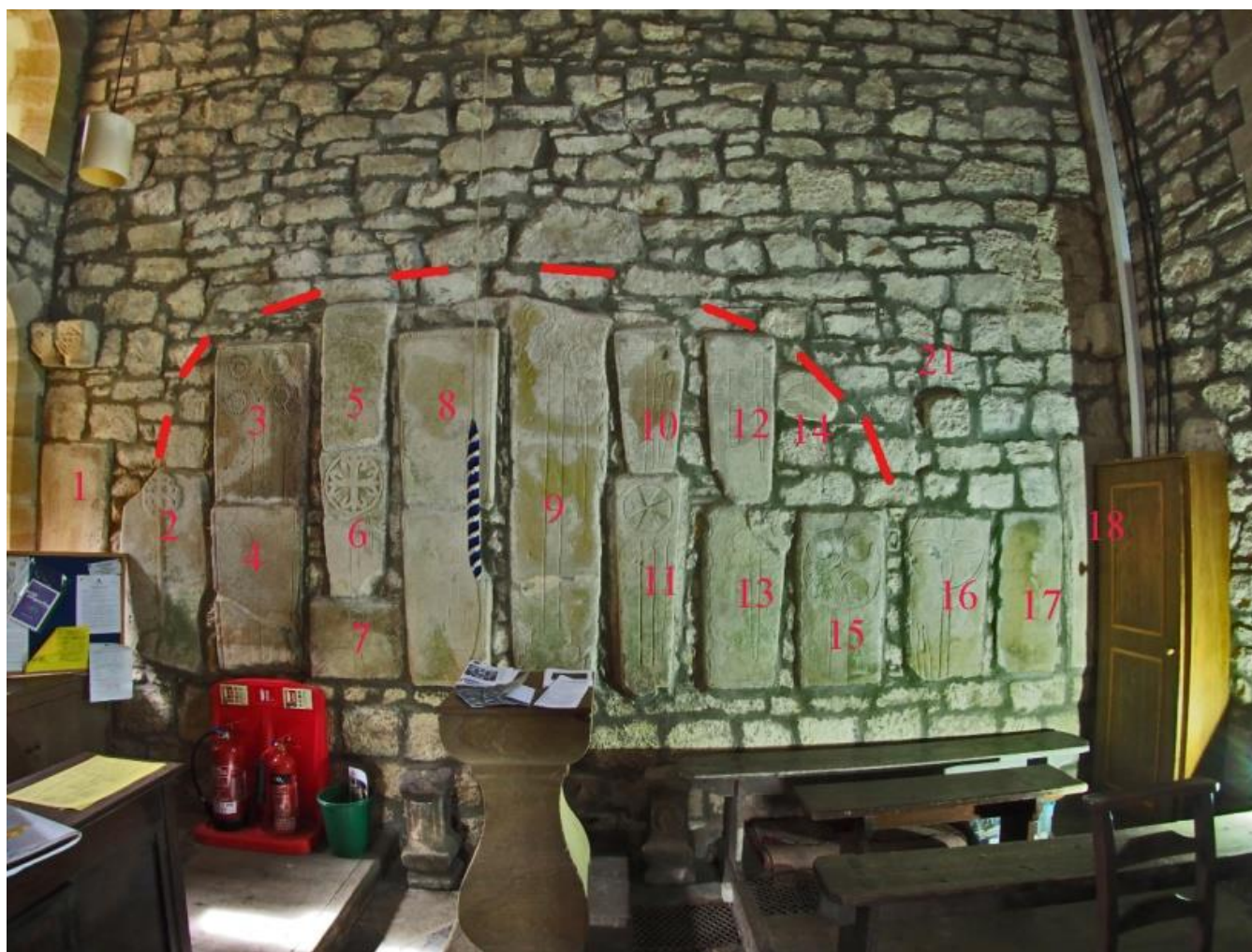
The re-set cross slabs (numbered), and possible vault line marked in red
