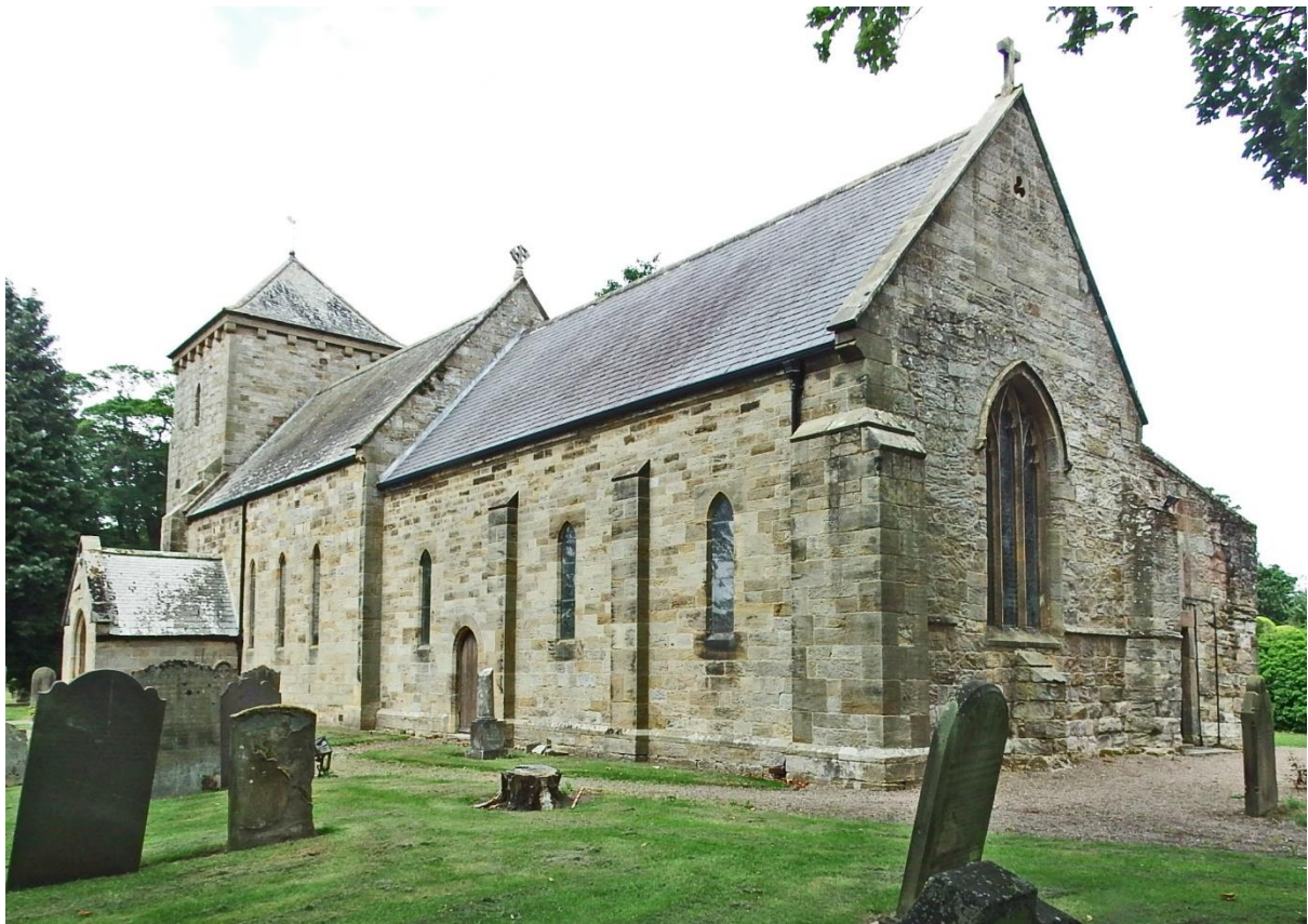
The church from the south-east
