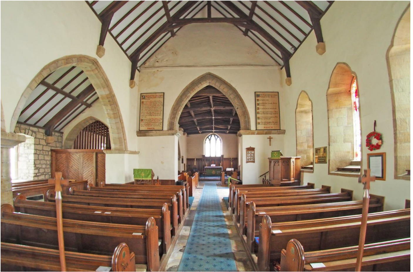
Interior looking east
