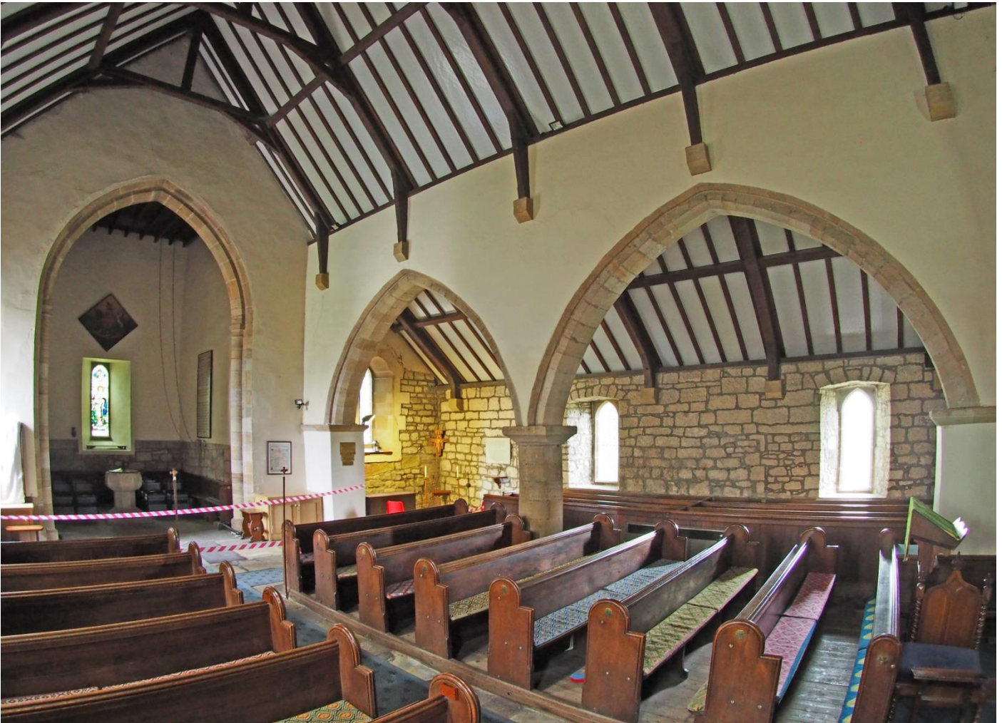
The nave looking north-west
