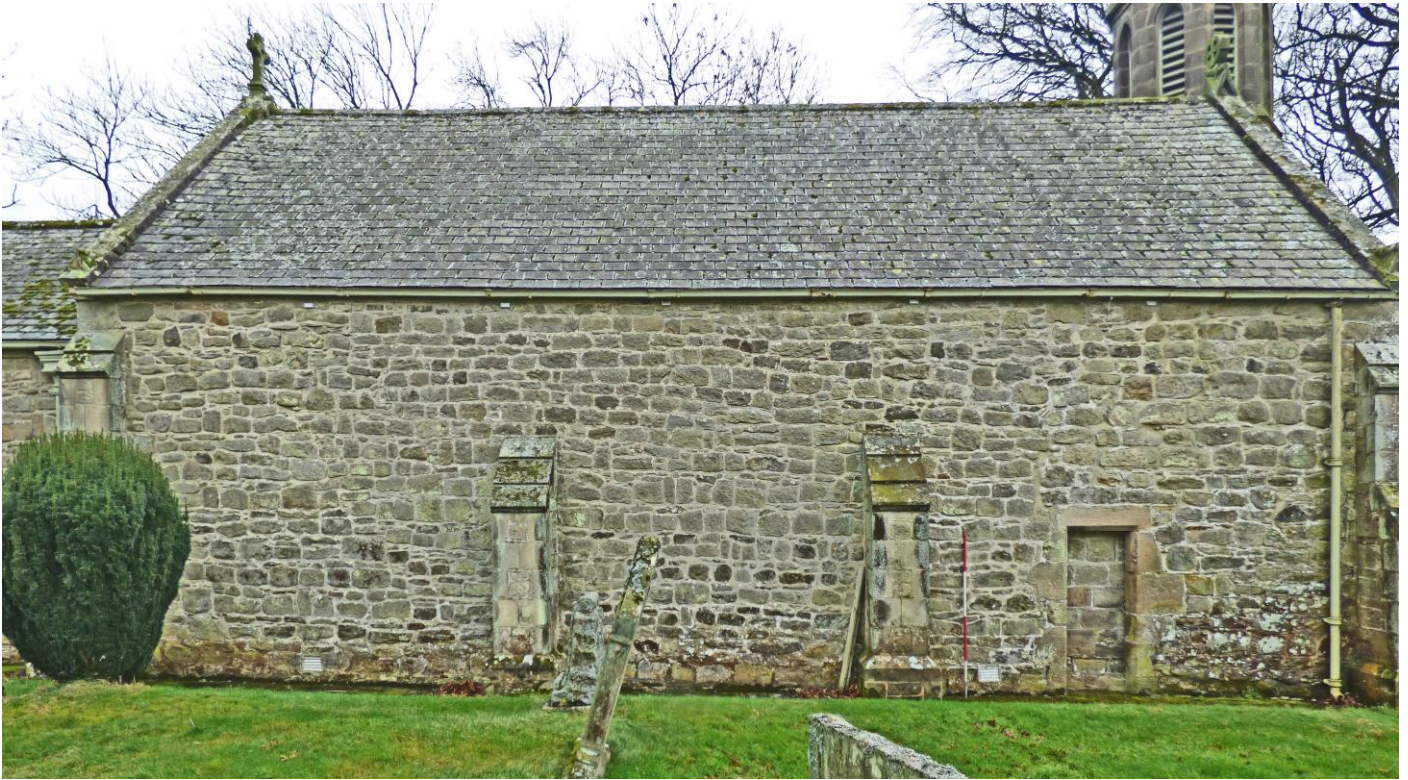
The north wall of the nave
