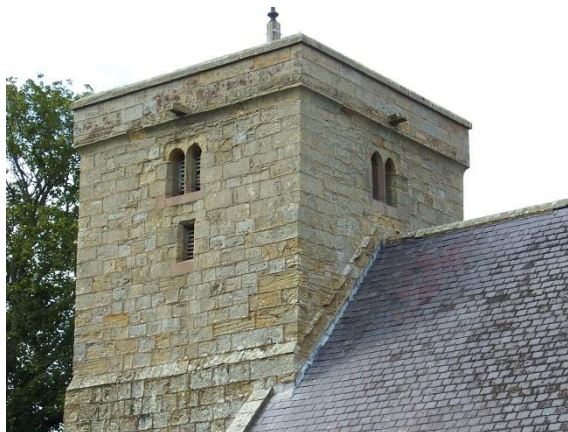
Tower from south-east
