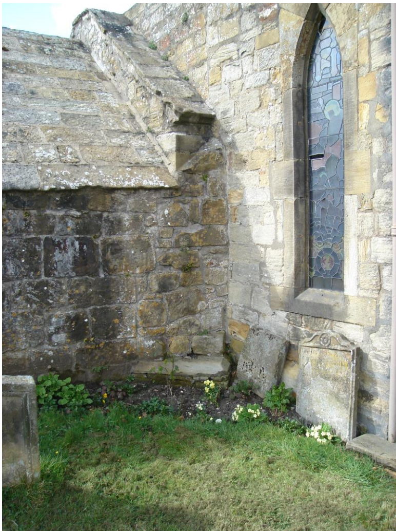
The east side of the south porch, showing the gabled front of the phase II porch behind its phase V successor. In the angle between porch and aisle wall is the base of the diagonal south-eastern buttress of the phase II porch. On the right is a mid-19 th century lancet window in the phase IV aisle wall.
