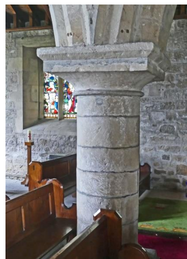
North arcade pier
