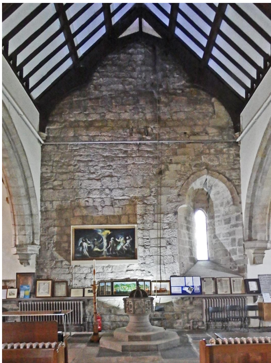
West end of nave
