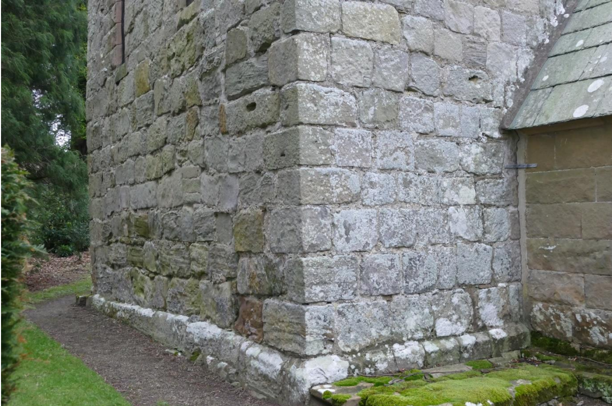
The south-west corner of the nave; contrast better-squared fabric of south wall (right) with less regular megalithic masonry of west end (left)
